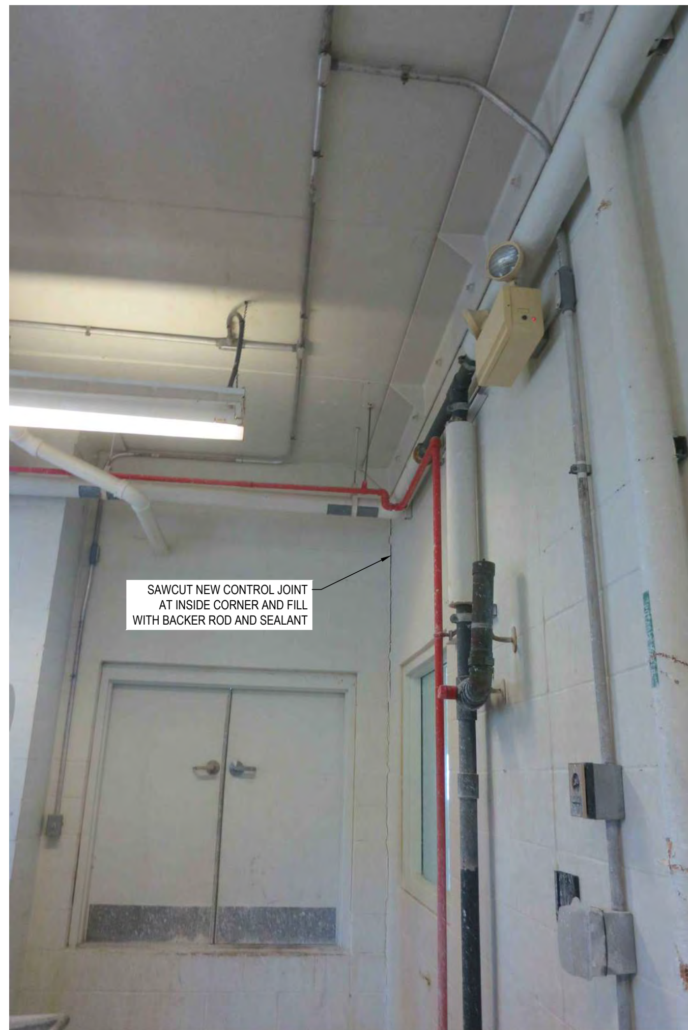
L INTERIOR NW CORNER OF LIME STORAGE ROOM S2.3 ORIGINAL SCALE: 1' = 1'-0"
