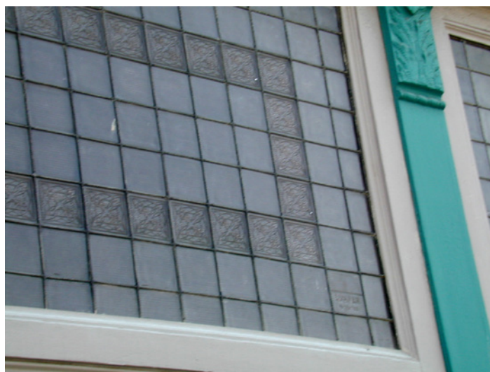
Prism glass was often used in transoms to direct light further into deep traditional commercial buildings.
