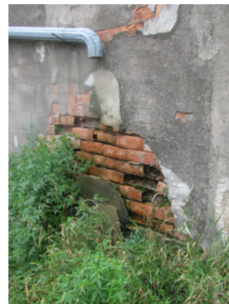
Deferred roof maintenance and improper downspouts can cause significant issues due to water infiltration.
