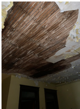
Deferred roof maintenance and improper downspouts can cause significant issues due to water infiltration.
