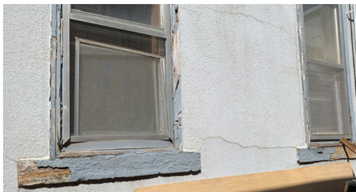
Deferred window maintenance is unsightly and can also affect the thermal performance of a building.
