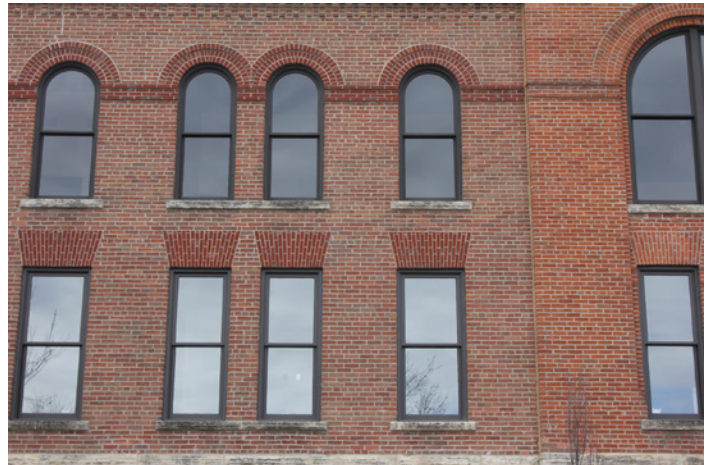
Appropriate window replacements fill the entire opening.
